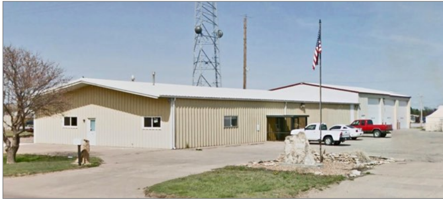
Russell County EMS and Extension facility
