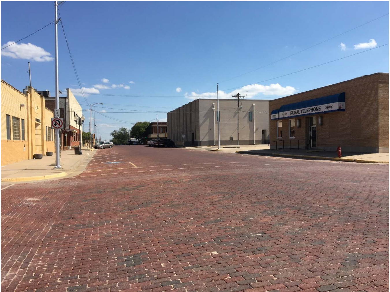
Figure 2: The existing street network is comprised primarily of concrete and brick streets. Brick streets are more prevalent in the downtown area, such as the brick street at 8 th & Maple Street.
